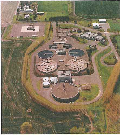
The McMinnville (Ore.) Water Reclamation Facility uses a pair of oxidation ditches to achieve biological phosphorus removal. The facility also uses chemical addition, tertiary clarification, and sand filtration to ensure that it meets its stringent phosphorus limit. City of McMinnville, Ore.
